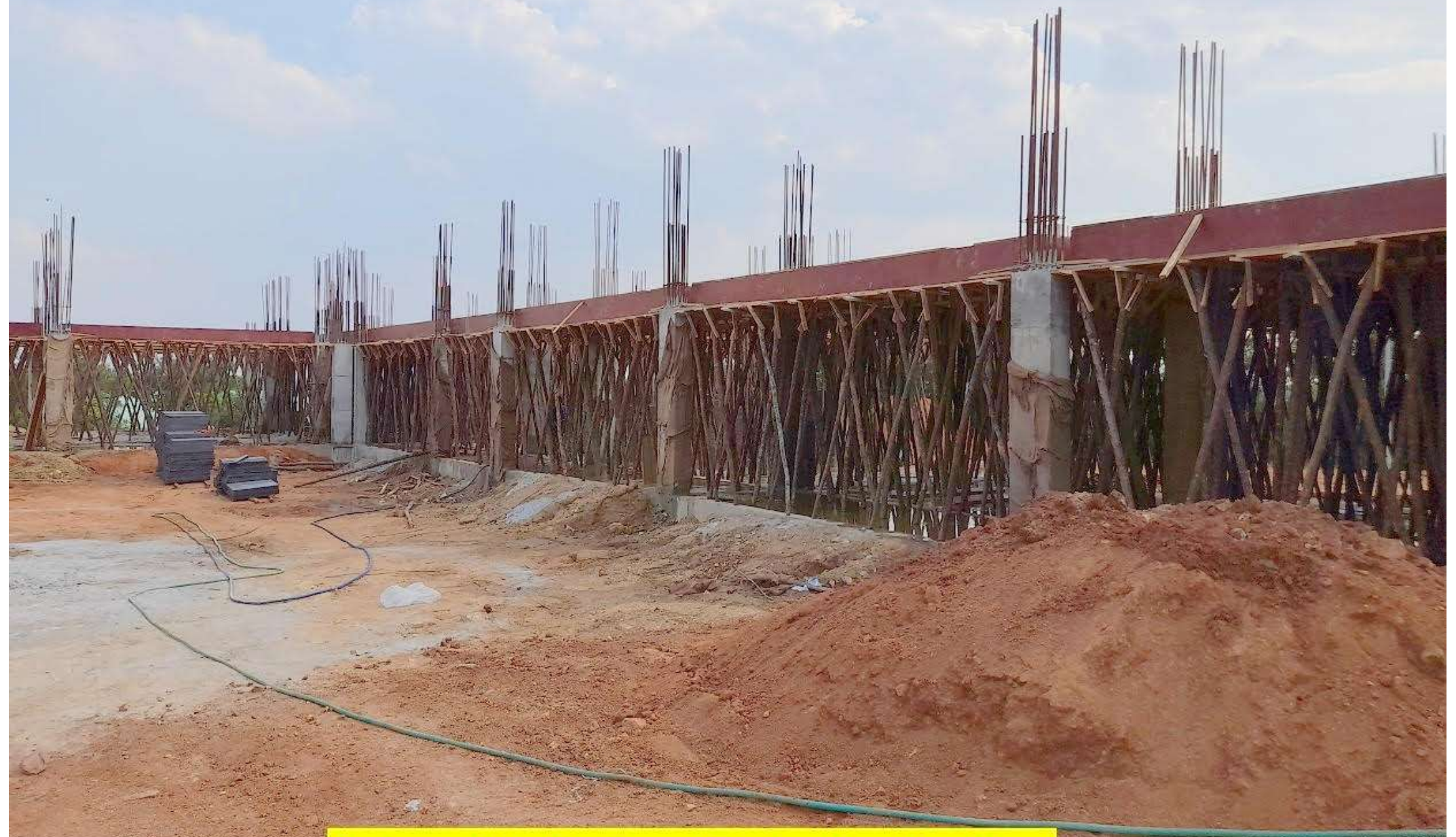
School Building-Slab shuttering
