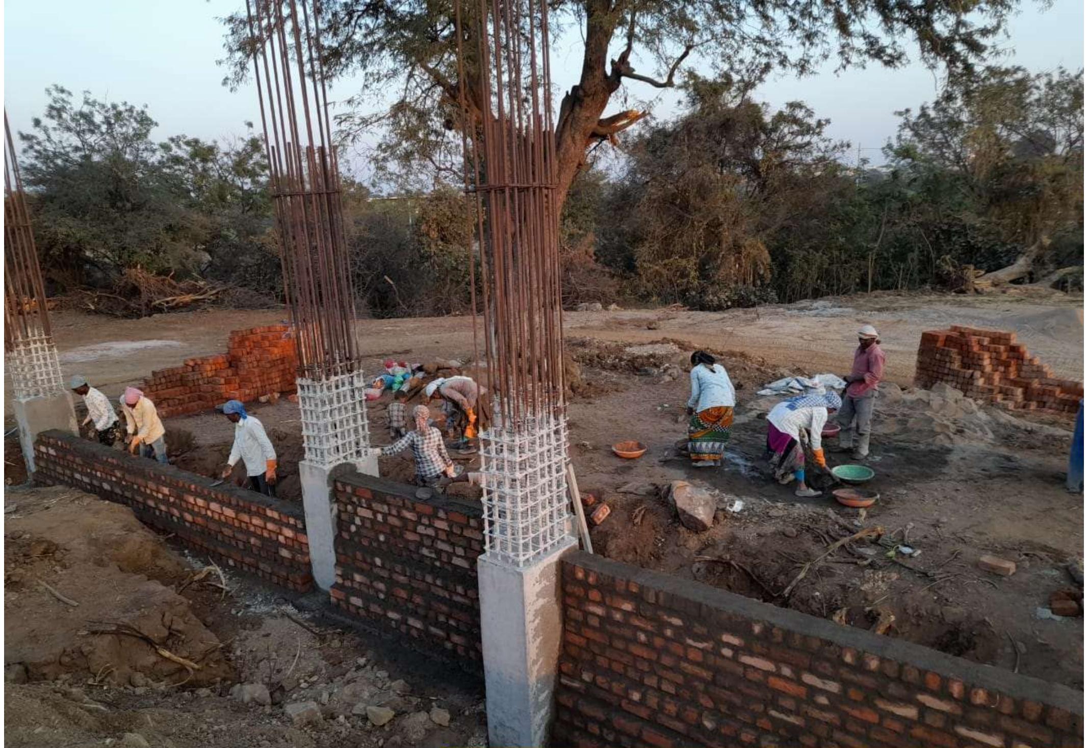
School Building-Outer Plinth
