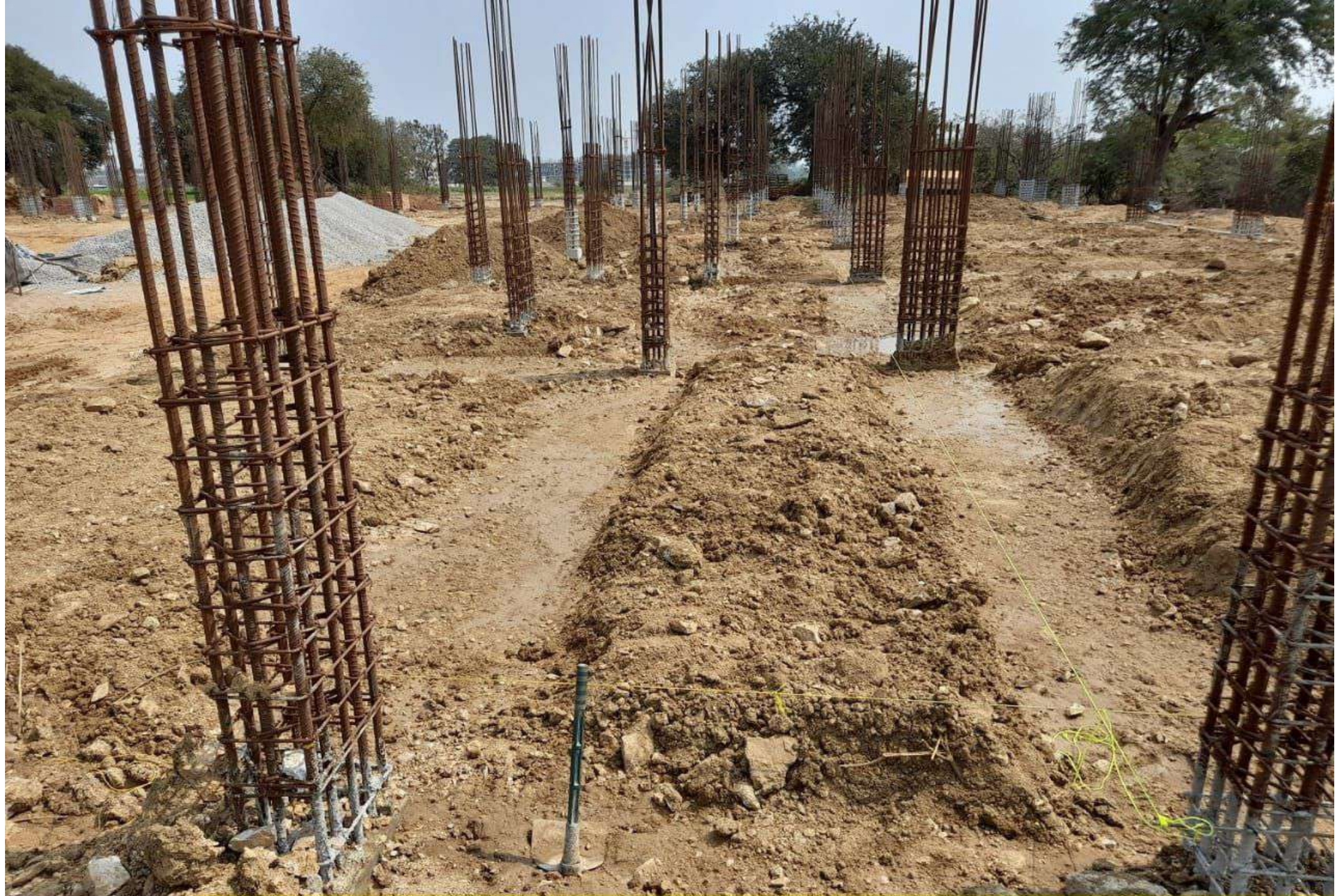
School Building...Layout for Plinth beam PCC
