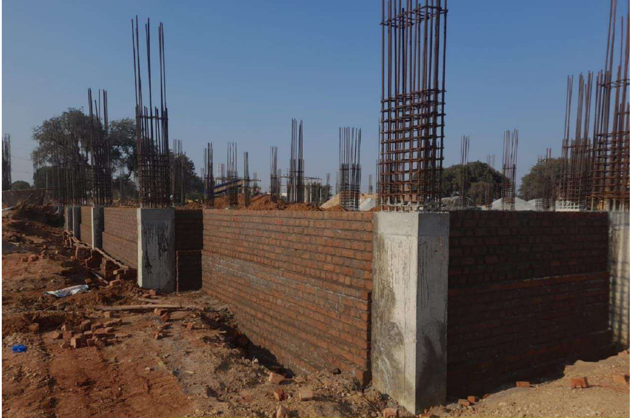
School Building-Plinth Brickwork at Back deep area
